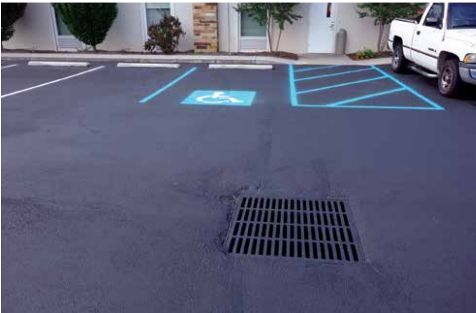
Figure 3. Freshly applied coal-tar sealcoat gives this parking lot a new look.
